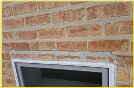
2.1 Unable to verify if a lintel is present
