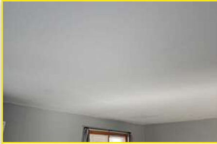
1.1 No switched receptacle found for lamp
