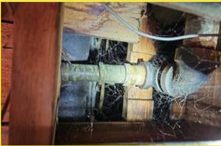
1.2 Going behind wall
