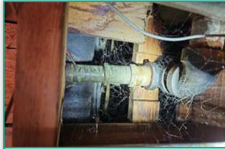
1.2 Going behind wall
